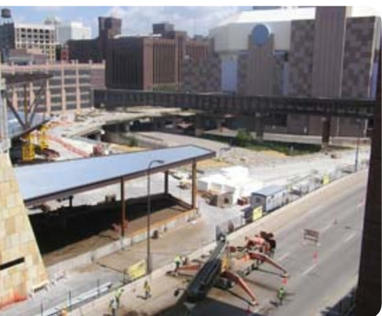
Retail store/plaza structure progress, July 25, 2008
