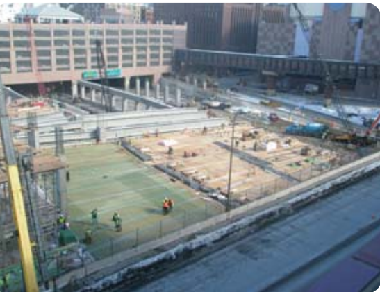
Retail store/plaza structure progress
