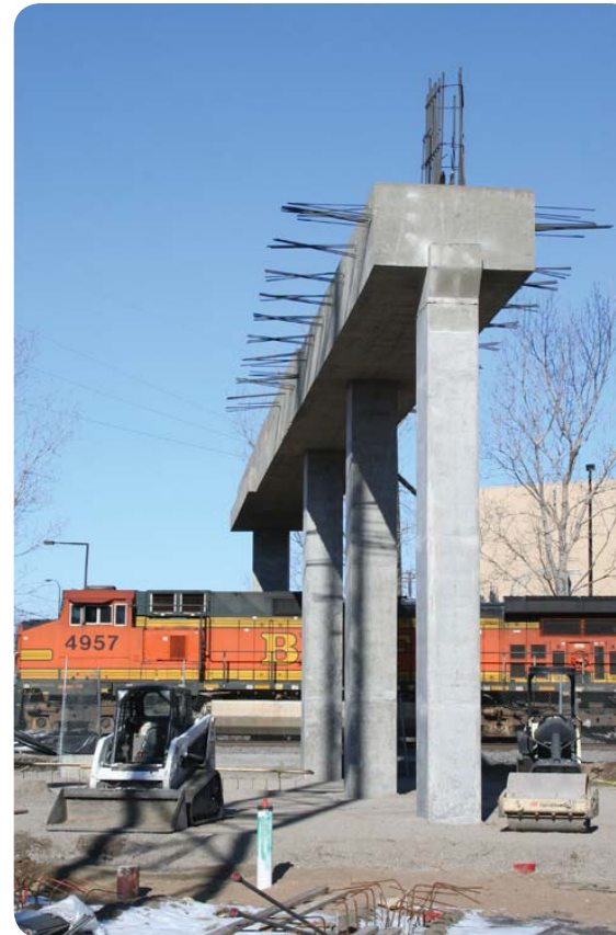
Cast in place girder over rail lines
