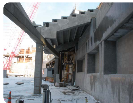
Service level looking north with overlook structure progress above
