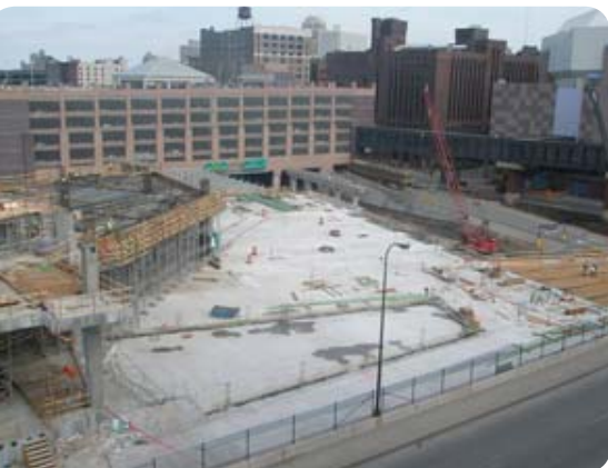
Retail store/plaza structure progress, April 9, 2008
