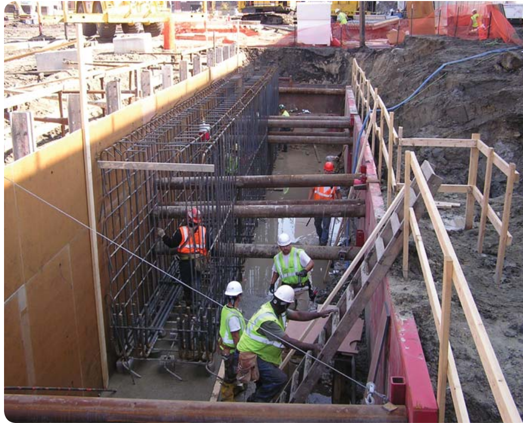
Transfer beam #11 in the field
