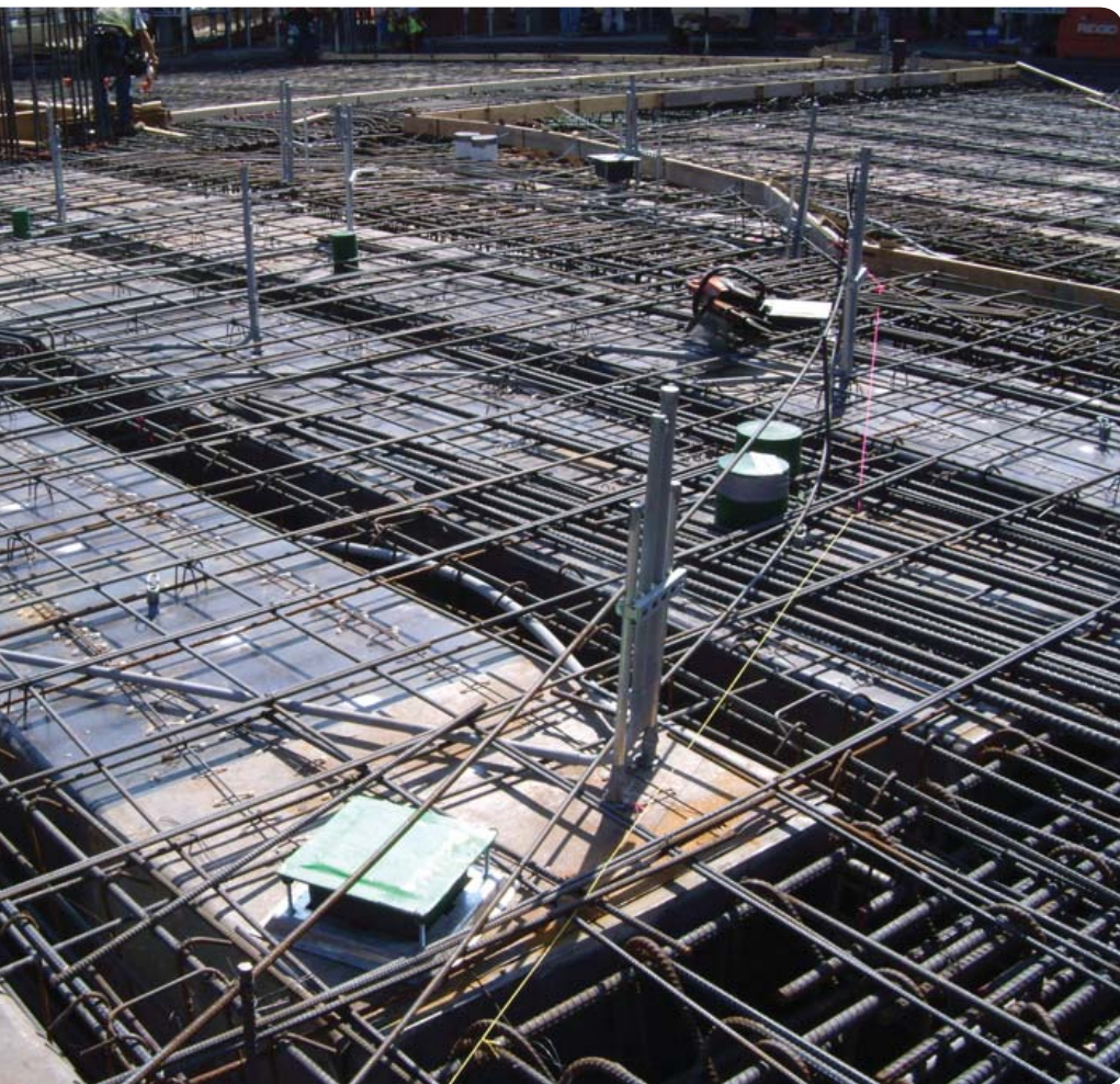
Main concourse pan and joist deck with reinforcing and sleeves
