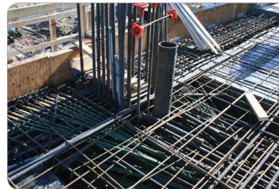
D-line column in the field with pipe penetration
